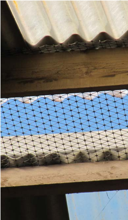
Bird proofing on an open ridge
