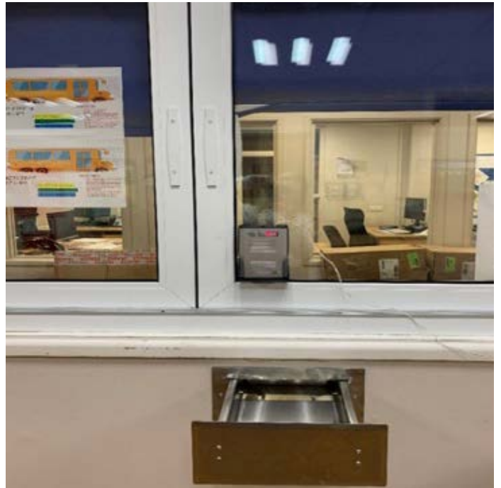
Figure 2. Example screened reception area and transfer drawer
