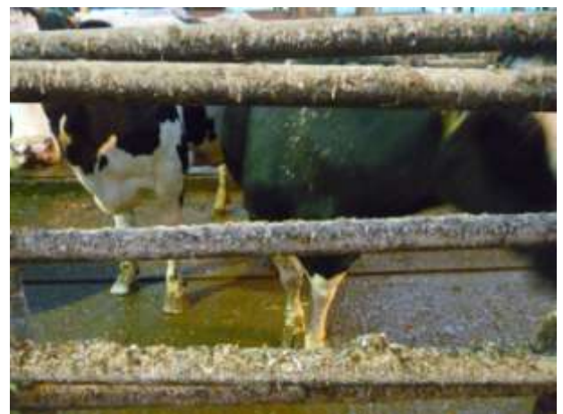
Plate. Accumulated fouling on rails in cow building
