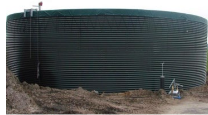
Lined corrugated panel store
