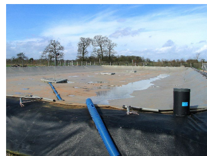
Supported slurry bag
