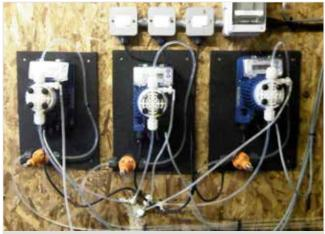
16. Sodium hypochlorite liquid injection using a metering pump at New Forest Fruit Company
