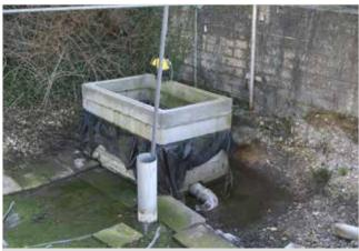
43. Silt trap prior to gravel bed
