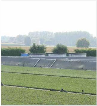
12. Slow sand filter installed at tray plant producer Avoird Trayplants in the Netherlands. The filter is contained in the left of the three tanks – the two tanks to the right are used for treated water
