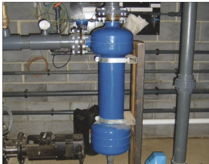
6 Centrifuge units are suitable for removing particles of sand, silt and clay from water intended for crop irrigation
