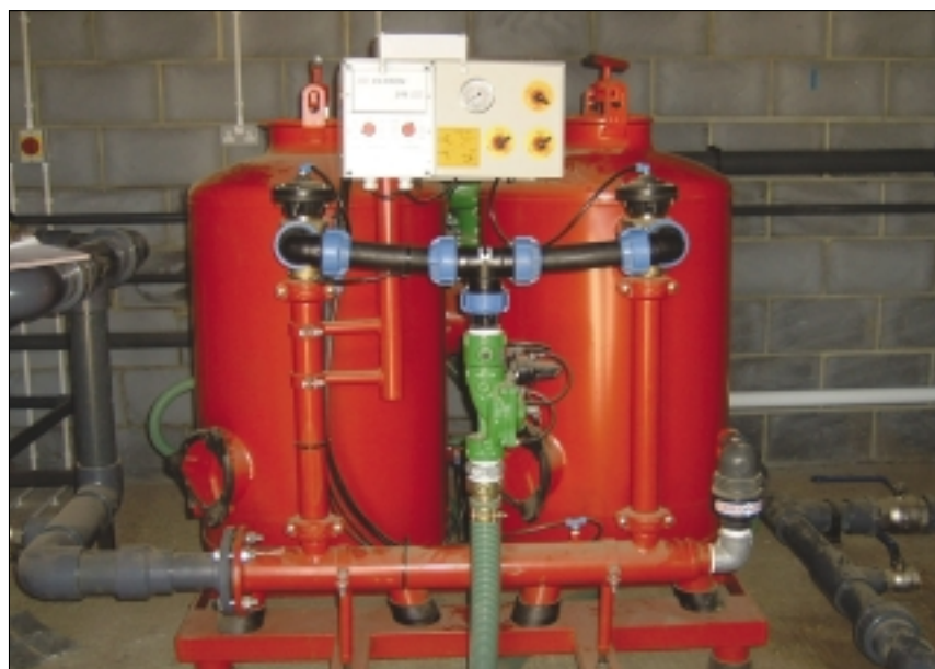
7 Graded sand filters are an effective way of removing larger biological contaminants from water
