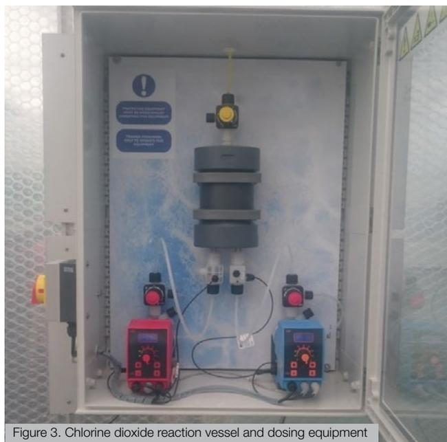
Figure 3. Chlorine dioxide reaction vessel and dosing equipment
