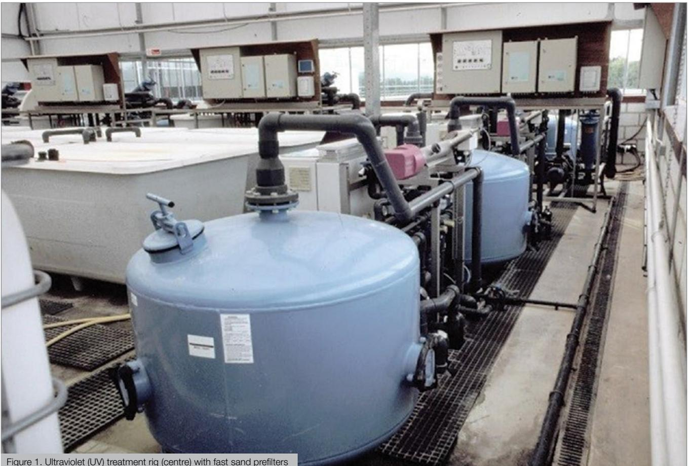
Figure 1. Ultraviolet (UV) treatment rig (centre) with fast sand prefiltration
