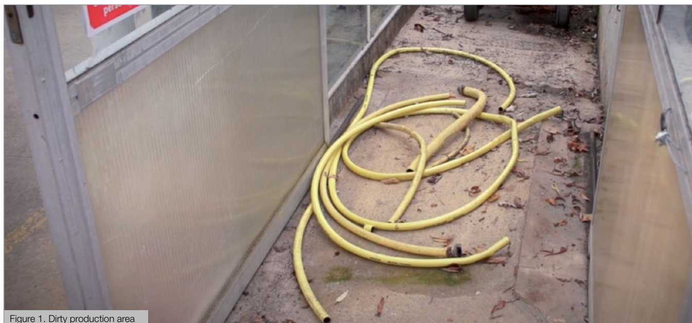
Figure 1. Dirty production area
