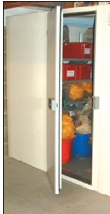
Fig 3 Purpose built cold store – expensive to construct but generally more suited to the storage of plant material
