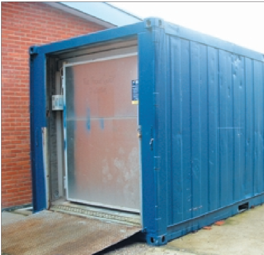
Fig 2 Modified refrigerated lorry body suitable for low temperature storage of bedding plant plugs – inexpensive to install but can dry plant material depending upon the speed of air movement in store
