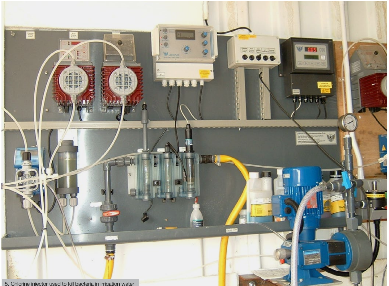
5. Chlorine injector used to kill bacteria in irrigation water
