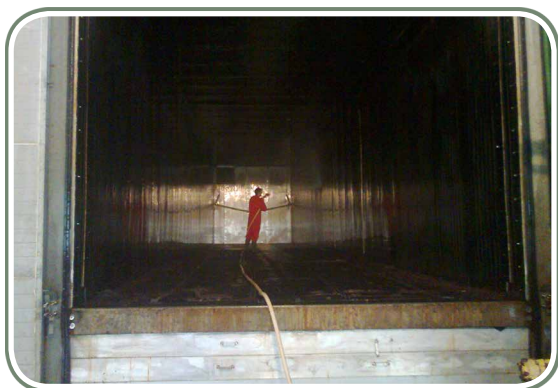
9. Phase 3 tunnel being cleaned post emptying
