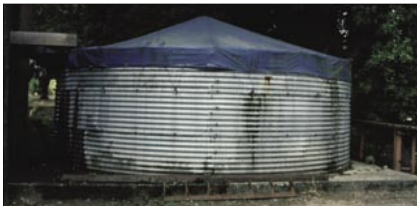
9 Cover water storage tanks to keep out dust and debris; contamination of irrigation water by Phytophthora or Pythium may lead to widespread root disease outbreaks on a nursery
