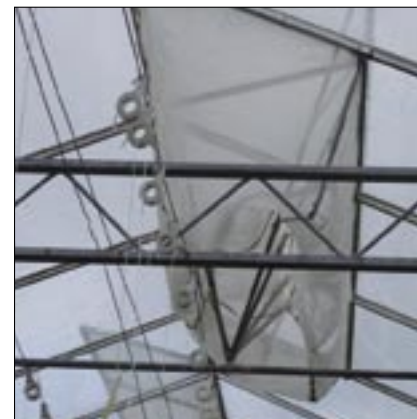
8 Netted vents can be used to exclude flying pests from high-health status areas, though fans will be required to ensure adequate air exchange
