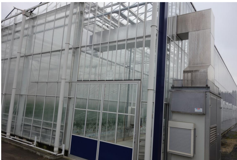
Figure 14: Incoming air heated through a heat exchanger
