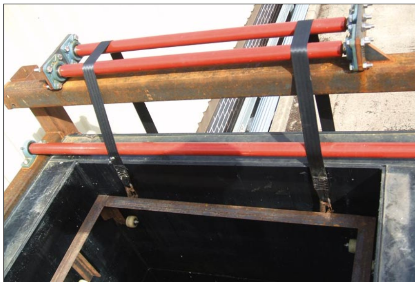
3 Platform fitted to top of tank to lower crates into tank
