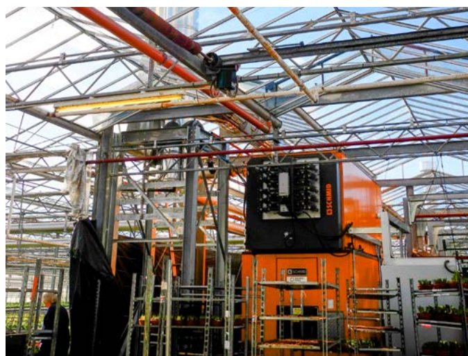
Figure 36. Biomass boiler
