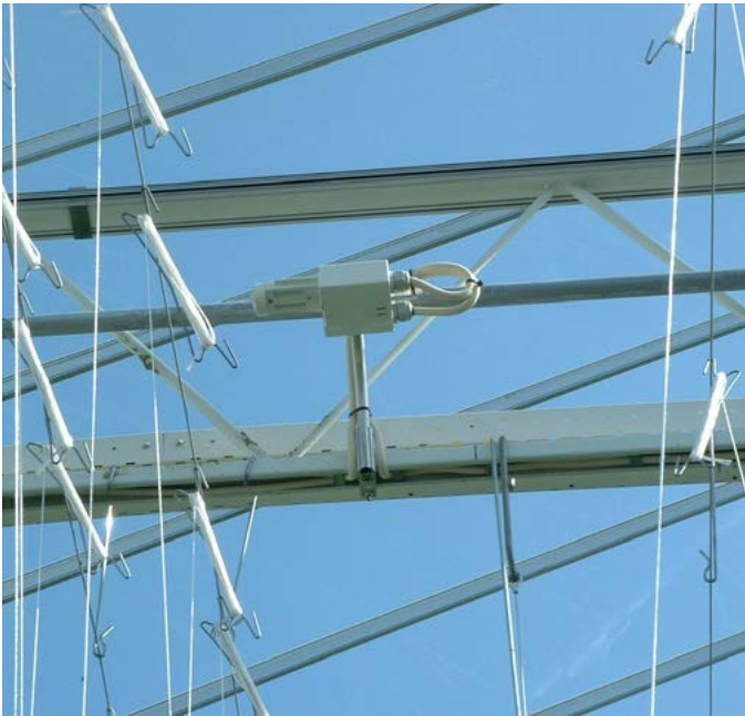
Figure 16. If at all possible, remove the lamp, reflector and electronic luminaire in summer to reduce crop shading
