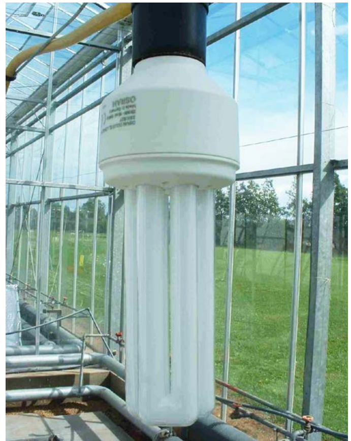
Figure 21. Compact fluorescent lamps can be effective sources of photoperiod lighting for some species
