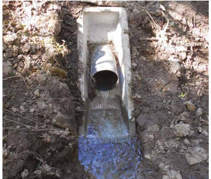
Figure 38. Precast concrete headwall (type K)
