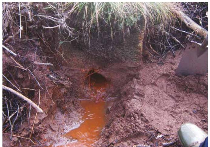
Figure 21. A blocked outfall can often be cleared in a matter of minutes with a spade
