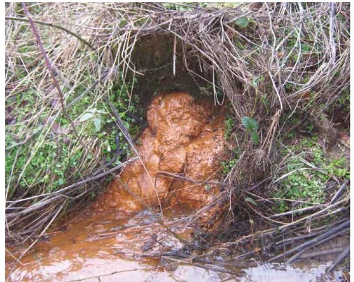
Figure 24. Drainage outfall blocked by ochre
