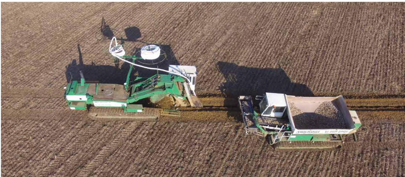
Figure 28. Installing land drains and stone backfill
