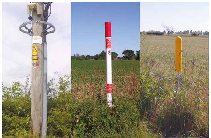
Figure 18. Signs indicating potential underground hazards
