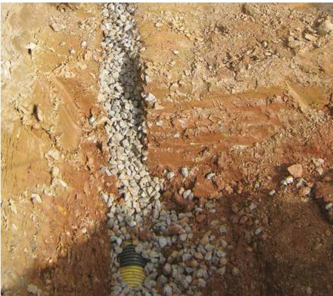
Figure 37. Washed gravel permeable fill over drain
