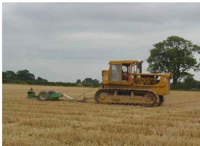
Figure 30. Installing mole drains
