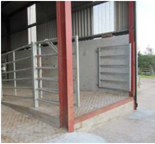
Loading ramp with height suitable for both trailers and HGV
