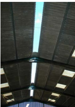
Ridge capping has been removed on this shed to allow stale air to escape
