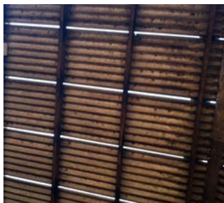
A slotted roof is good where animals are housed all year
