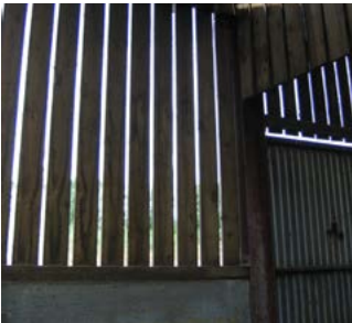
Space boarding with a simple additional inlet area allows fresh air to enter
