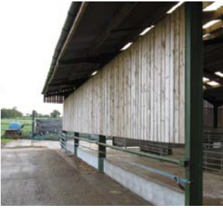
Space boarding with simple additional inlet area above
