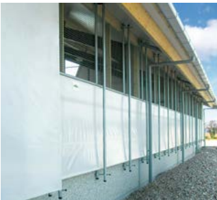
A ventilated roller blind offers protection against draughts
