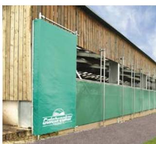
Moving curtains provide flexible inflow of fresh air
