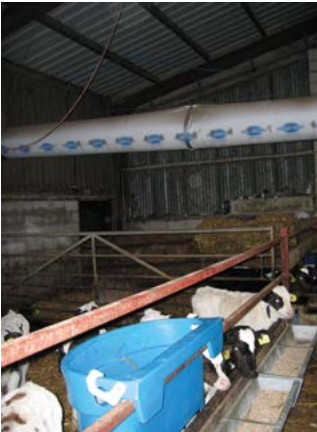
Positive pressure ducting in a calf house
