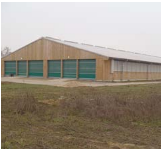
Modern cattle building with a large area of diffuse inlets
