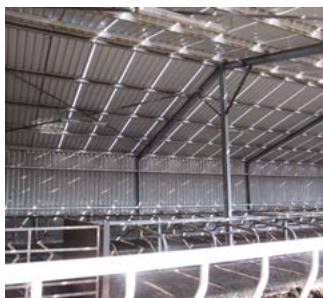
Slotted roof made of fibre cement profiled sheeting
