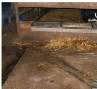
Cutting channels into the existing floor can improve drainage
