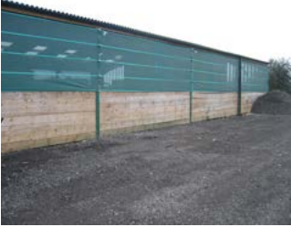
Timber sidewall with ventilated cladding delivers clean, fresh air into the building
