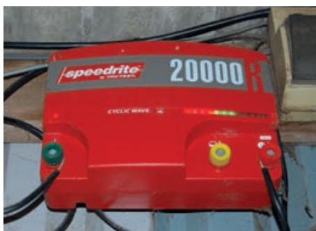
The energiser is the powerhouse of the electric fence
