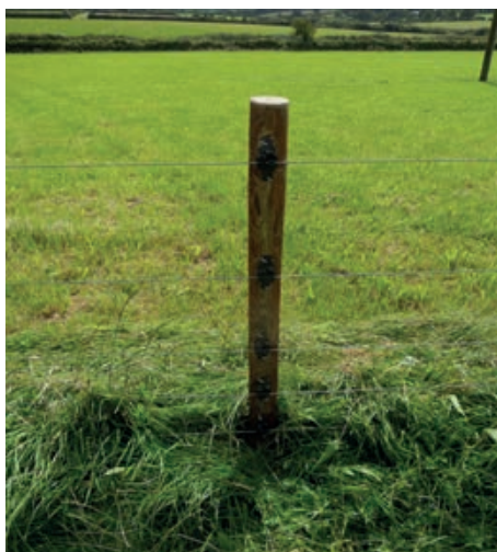
Creosoted wooden stake and 5 claw-type insulators with high tensile 2.5mm steel wire
