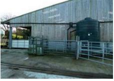
Gravity above ground storage with filter unit at top left (courtesy of ADAS)
