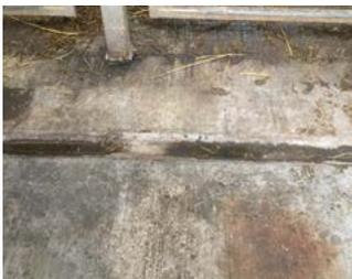
A simple drainage channel removes excess water away from the calves
