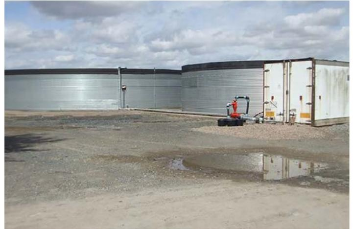
Figure 4. Water storage tanks can add to the short-term water supply resilience of a business
