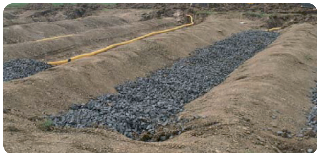
Figure 3: Base with ridges and permeable fill over drain pipes
