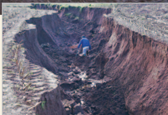
Serious gully erosion
