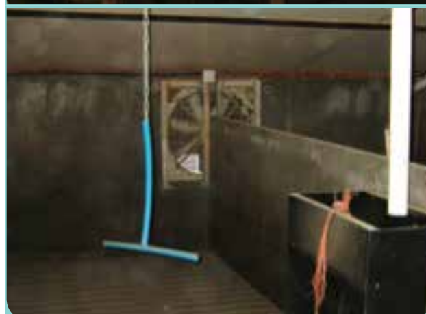
Internal views showing the centre passage and pen layout (top), the inlets above the passage (middle) and the fans low in the outer walls at the back of the pens (bottom)
