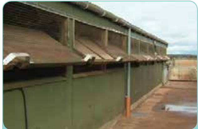
ACNV side-to-side building showing the wall vents
