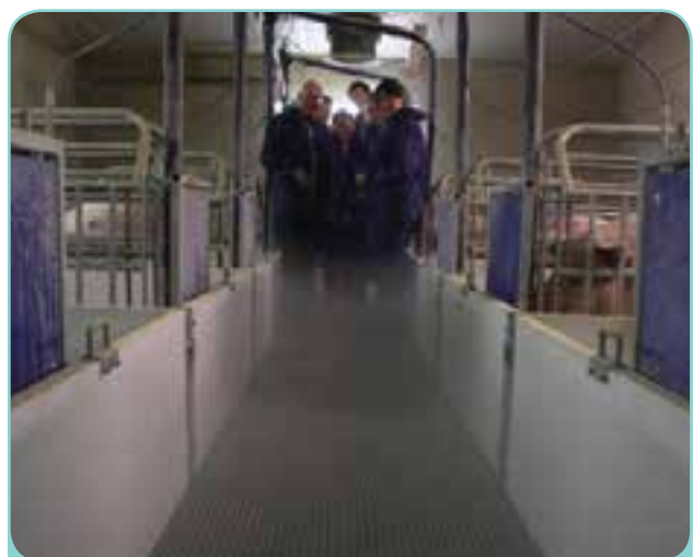
Under passage ventilation system
