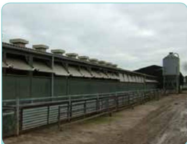
A modern, side-to-side, ACNV building with ridge outlets
