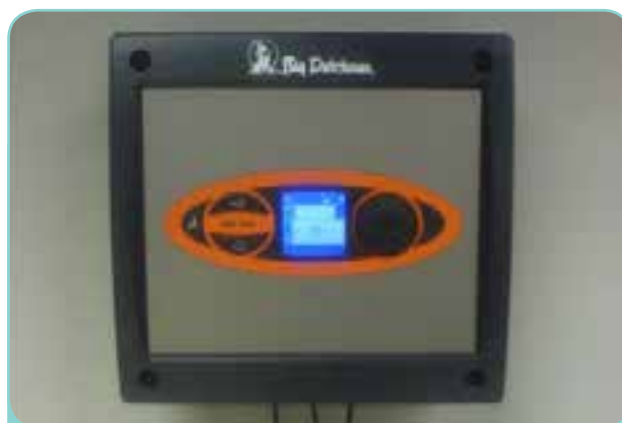
Ventilation control computer
