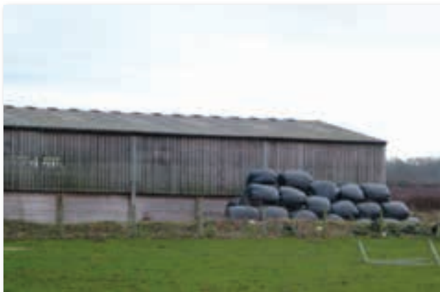
A naturally ventilated general purpose building
