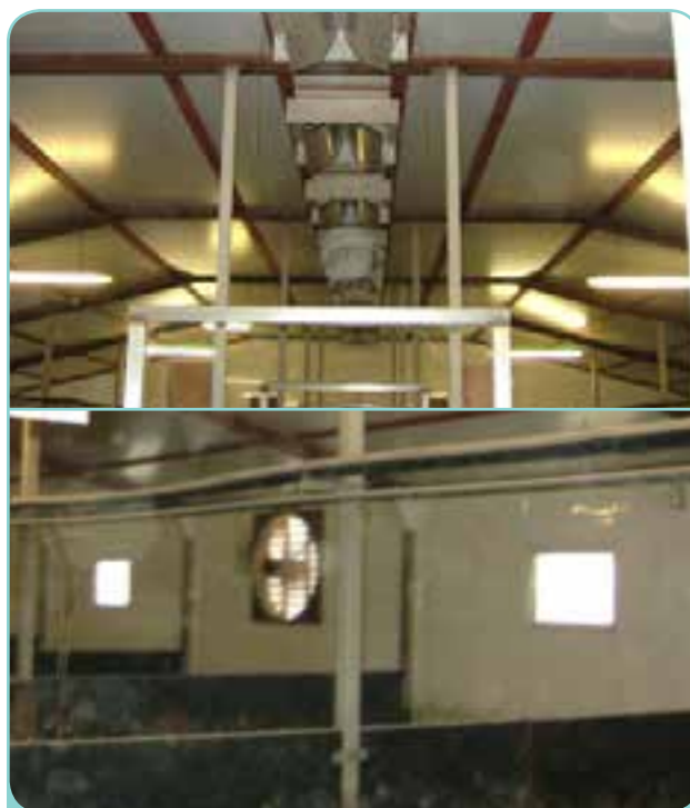
Pictures showing ridge inlets (top) and side extraction (bottom)
