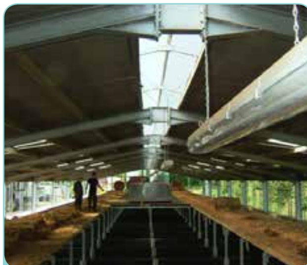
Internal view showing the two walkways, the side curtained openings and the open ridge
