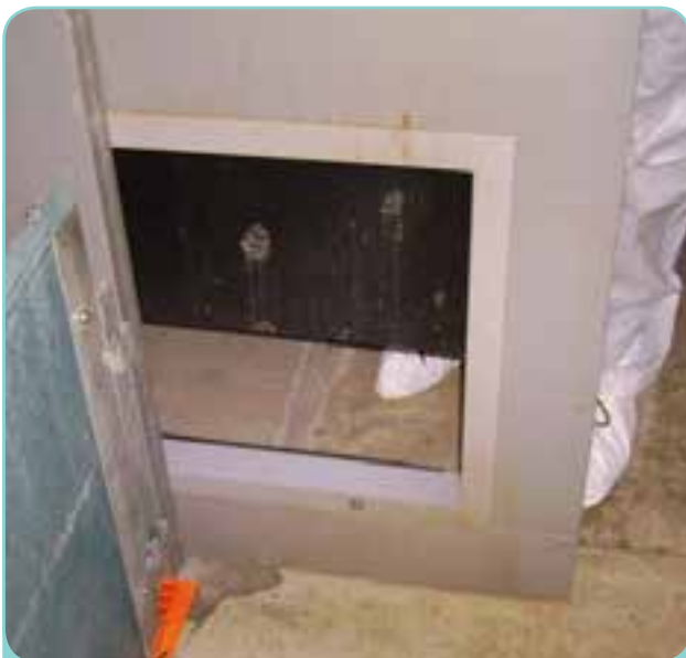
A door ventilation opening
