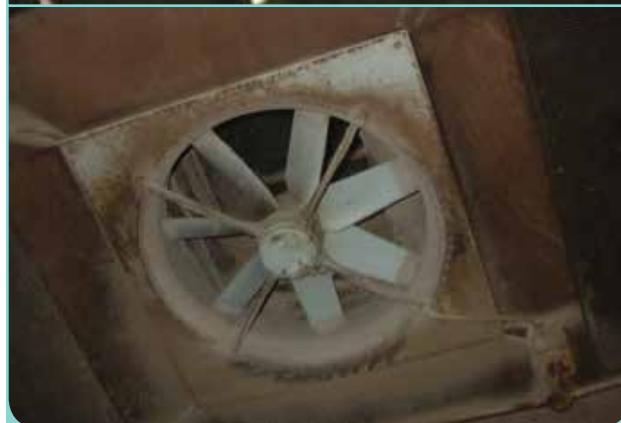
Interior view of the pens showing the hand operated vents at the back of the pen and the feeder (top) and the fan in the ceiling (bottom)
