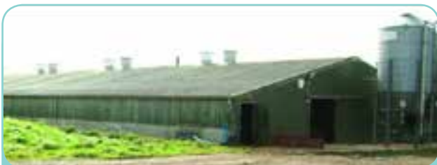
View of the building showing the fan chimneys for the six rooms accessed from the passageway running down the side
