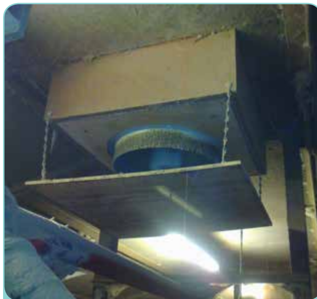
Pressurising fan with a spreader board beneath
