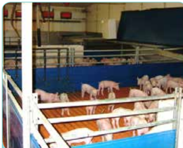
Interior of the building, showing the four pens to the right-hand side of the centre passage and the inlets in the side wall
