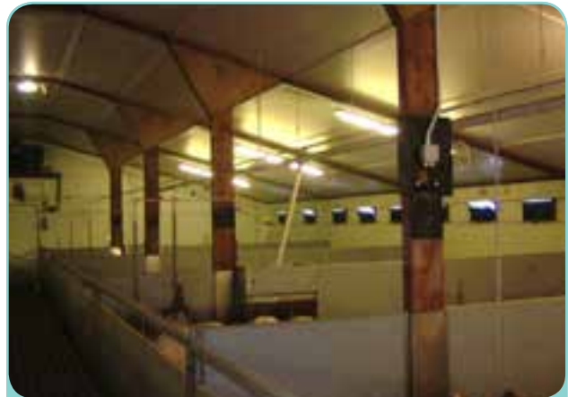
Photo showing side inlets for ridge extraction
