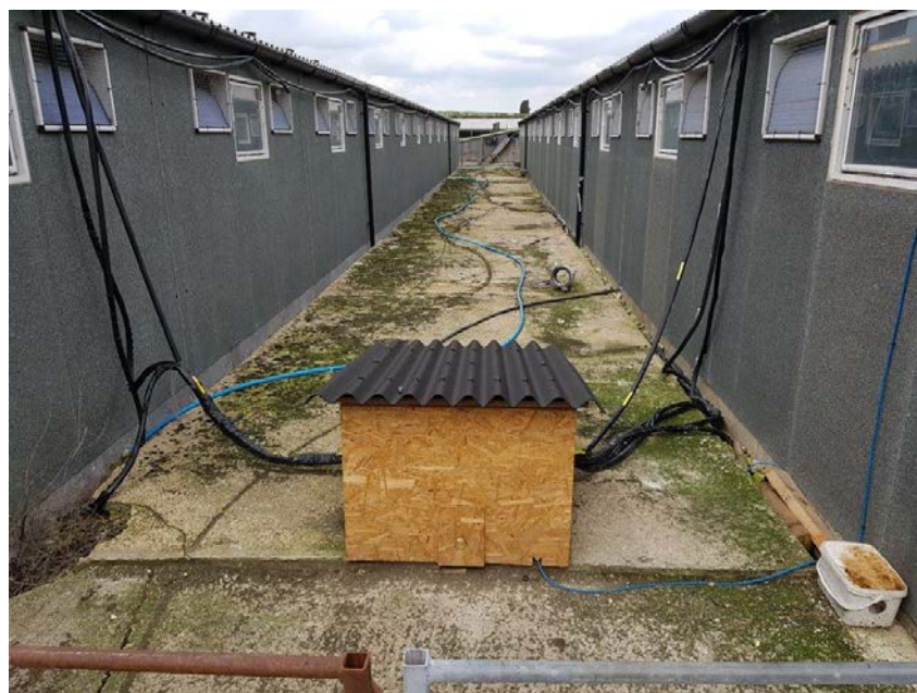
Photo 1: Area between two buildings to place ammonia analyser
