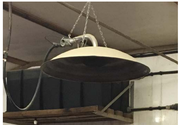
Figure 71. Gas plaque heaters are widely used for chick brooding
