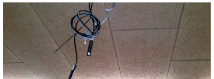
Figure 81. Humidistat and temperature sensors during installation
