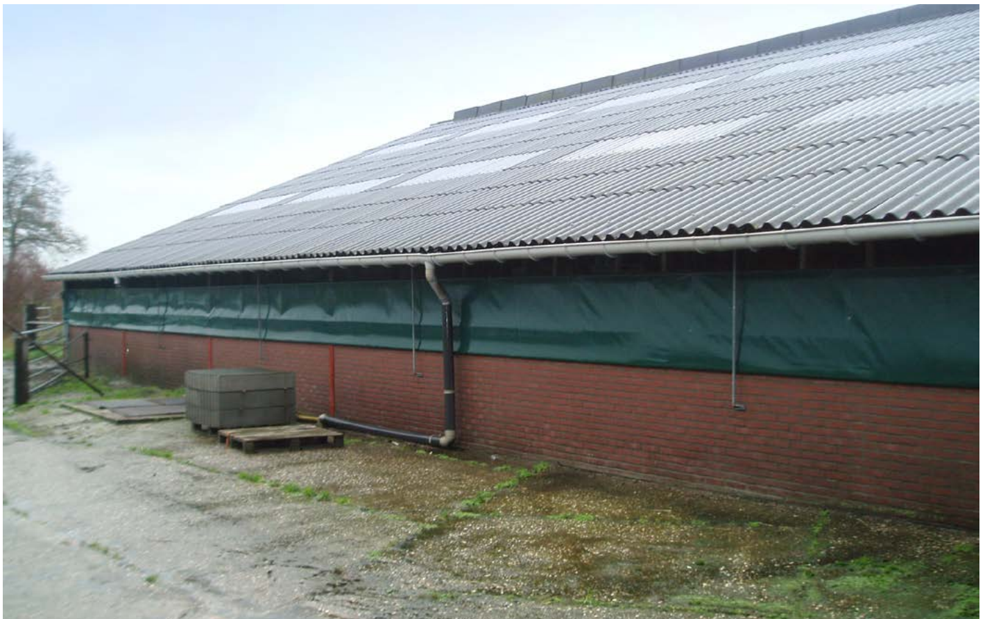
Figure 22. Cattle building with controlled natural ventilation via controlled side curtain inlets and an open ridge
