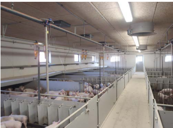
Figure 85. Lit weaner pig building with differentiated areas for lying, feeding and dunging
