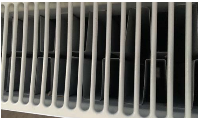
Figure 59c. Convective fins combined with water-filled radiator
