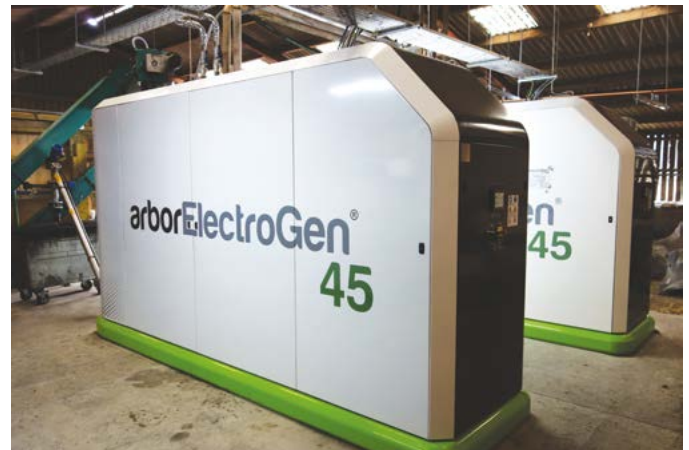
Figure 57. Biomass CHP
