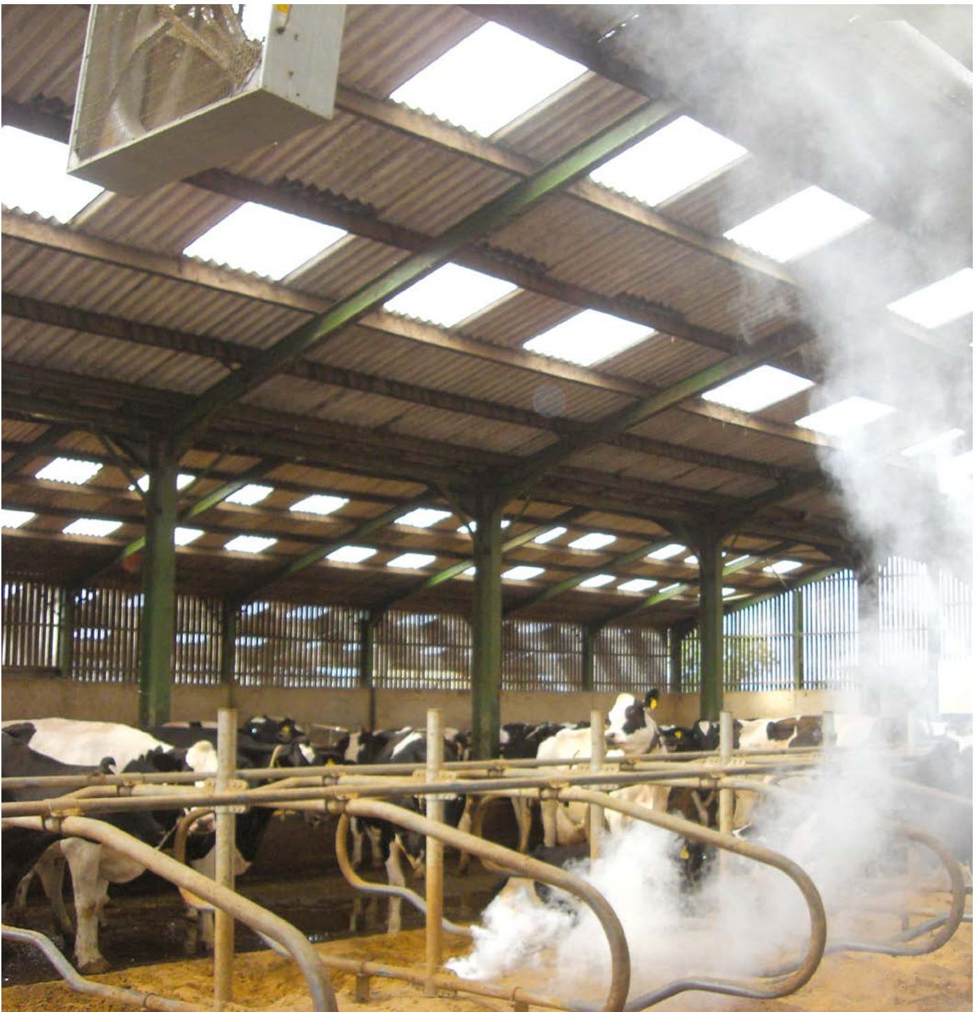
Figure 1. Confirming air movement using smoke
