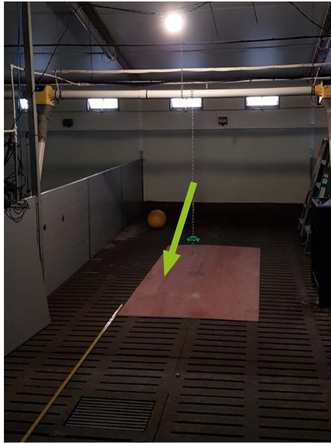
Figure 7. The test rig on a working pig unit, with a single ALIS lamp mounted at the recommended mounting height
