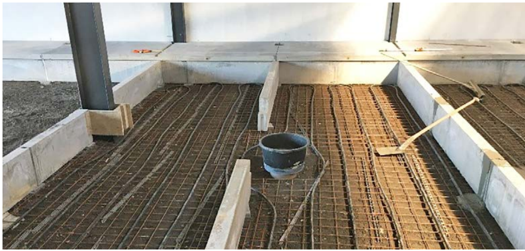
Figure 4. Cooling pipes laid out, wired to reinforcing mesh
