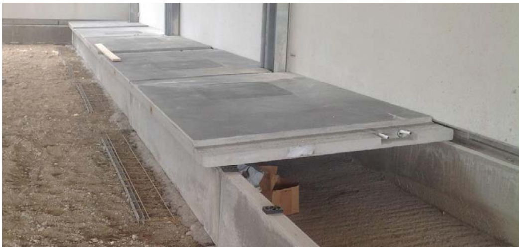
Figure 7. Heating pipes embedded in solid floor lying area over ventilation duct Image courtesy of AgriFarm Group
