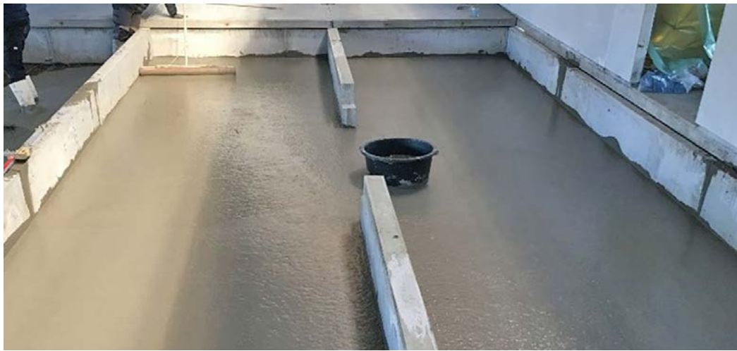
Figure 5. Cooling pipes buried under cellar floor
