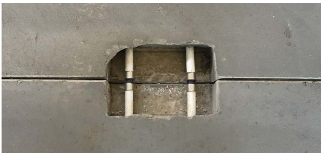
Figure 8. Heating pipes embedded in solid floor; jointing
