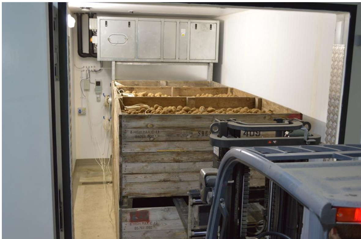
Fig. 1. Boxes stacked two high, three deep against a plenum, at the back of the store, for positive 'letterbox' ventilation.
