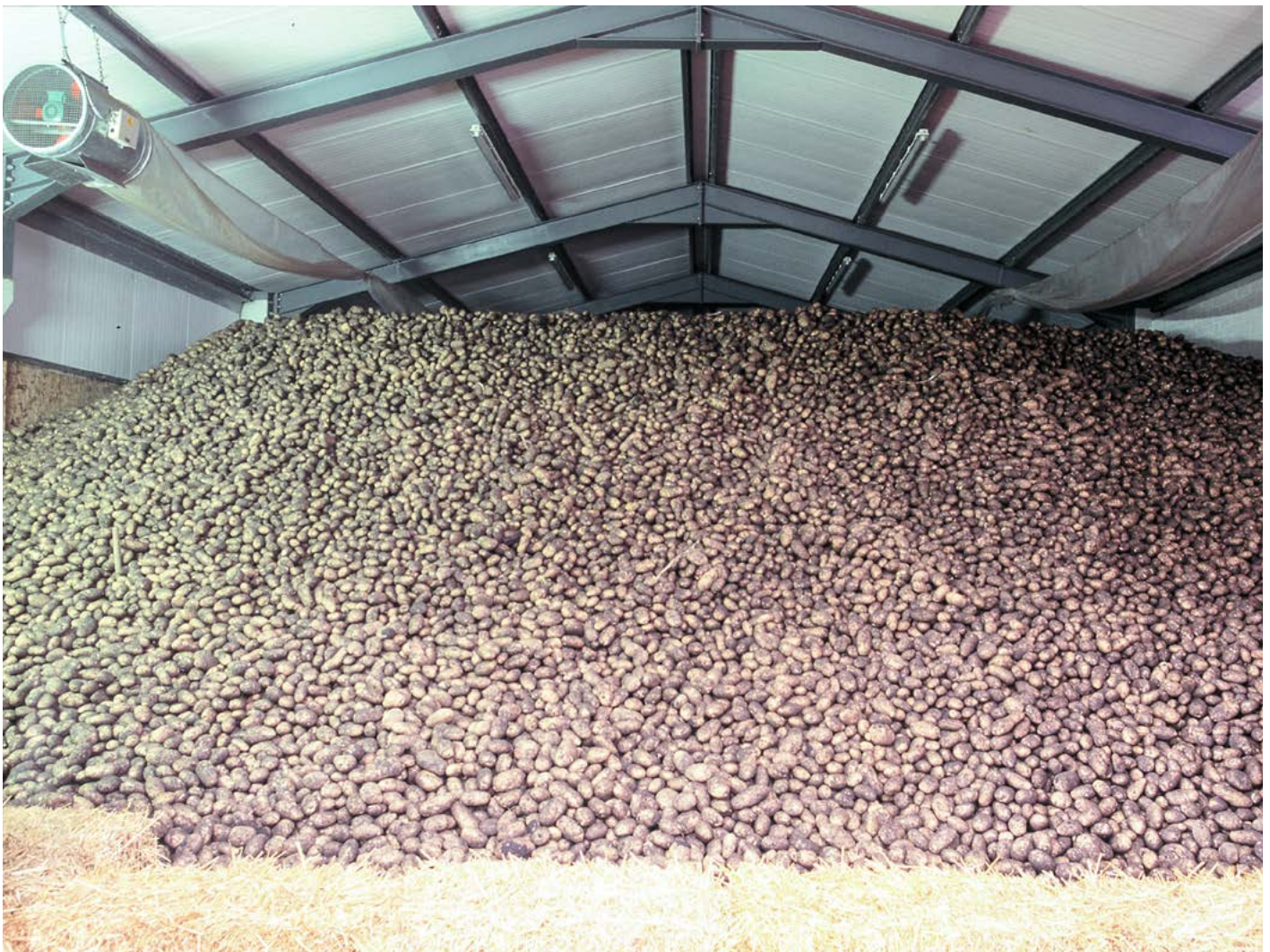
Figure 19. Roof-space heating in a bulk store
