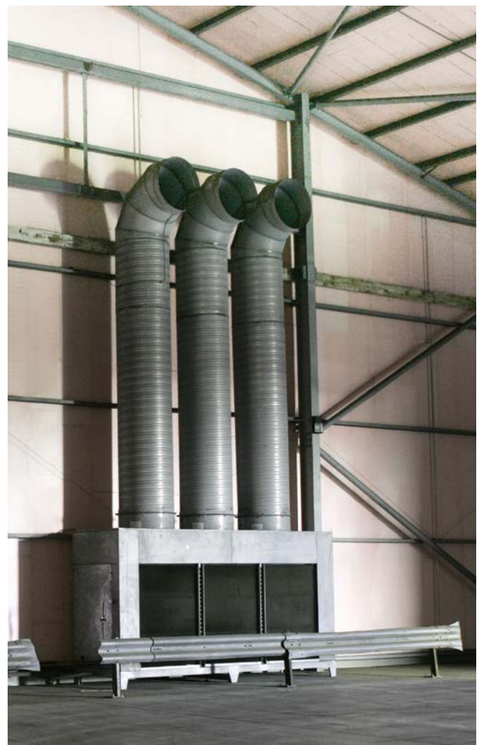
Figure 20. Floor-mounted fridge unit typical of older installations
