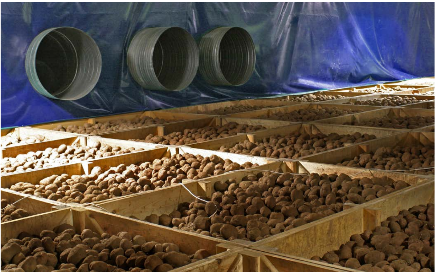
Figure 11. An air separator curtain boosts ventilation efficiency significantly by preventing short circuiting
