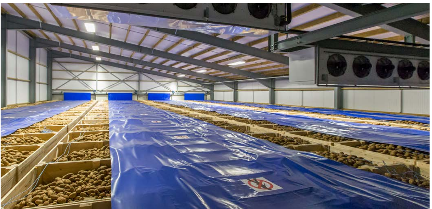
Figure 13. Lateral suction is a positive ventilation option for box storage
