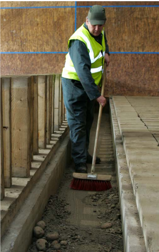
Figure 8. Remove all debris before loading
