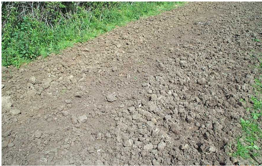
Figure 12. Close-up of surface of stabilised cow track
