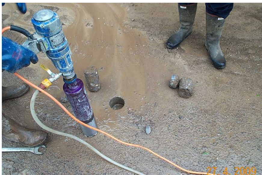
Figure 6. Coring equipment showing core removed
