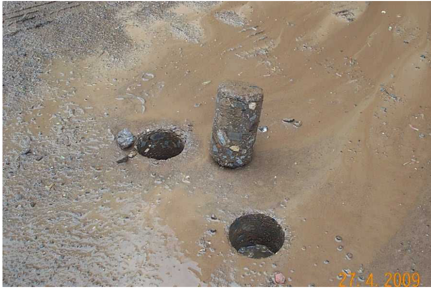
Figure 7. Core of stabilised soil material
