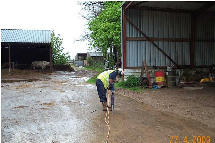
Figure 5. Coring at Warren Farm yard area
