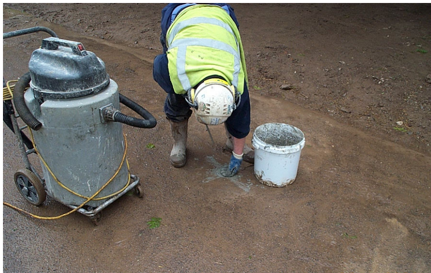
Figure 8. Vacuum used to clean out core holes prior to reinstating with concrete mix
