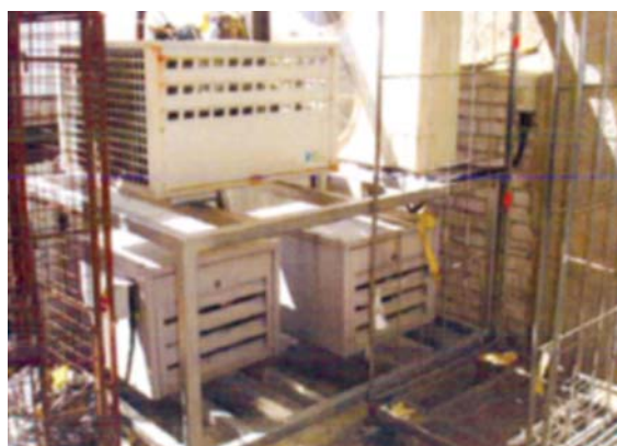
Condensers in direct sunlight, drawing hot air from its neighbour
