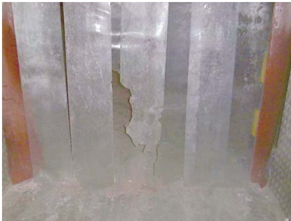
Strip curtains in poor condition
