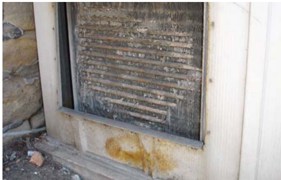
Condenser on the verge of failing
