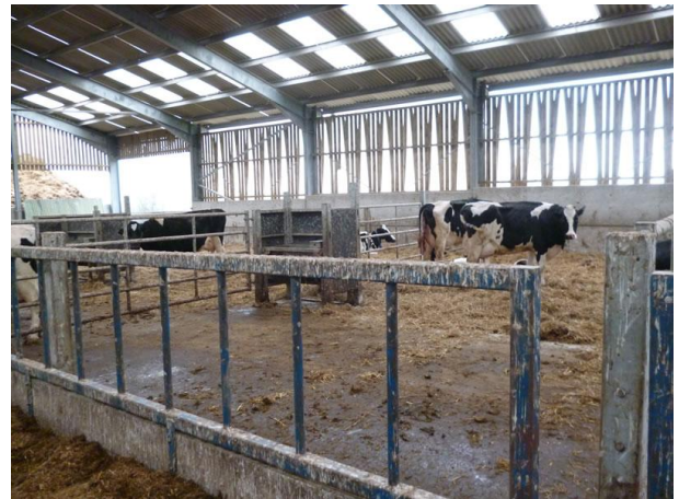
Fouling inside cow building
