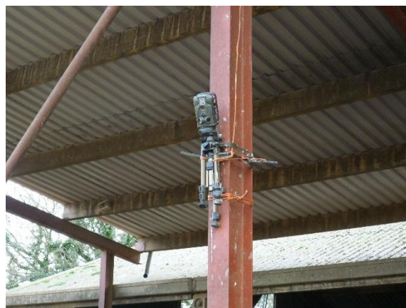
Plate 5 Timelapse camera set up
