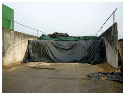
Plate 8 Netting to end gates (top), covered maize silage clamp
