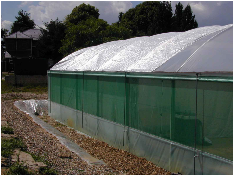
Plate 4. The twin-span polyhouse showing the external roof shade. Nylon monofil sewn into the edges of each piece of shade cloth and anchored to eyes in the gutters held the shade securely in place.
