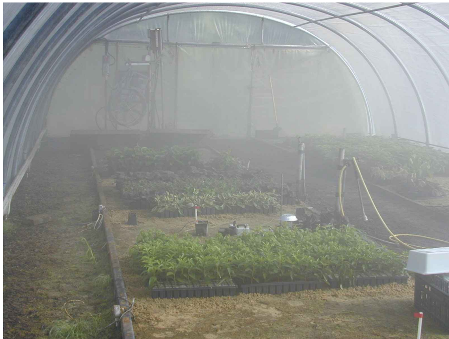
Plate 6. The ventilated fog house with fog lingering in the air about 10 minutes after the last operation of the fogger. The fogger is at the back left of the picture, with the air intake for forced ventilation immediately behind it.
