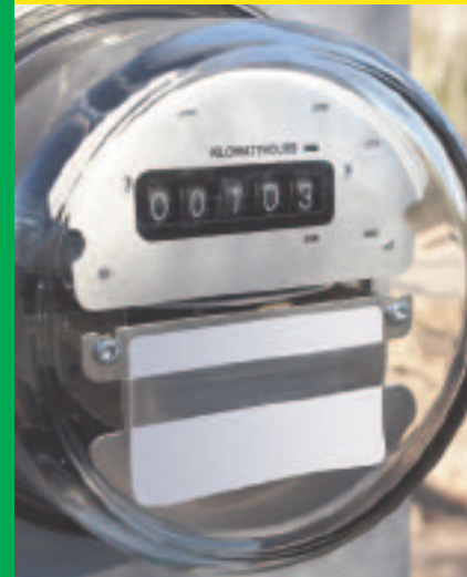
Install monitoring equipment
