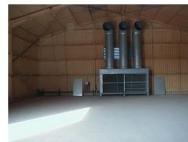
A store with non-positive 'overhead throw' air delivery system. CIPC applications in this store type are problematic and may be subject to stricter controls in the future.
